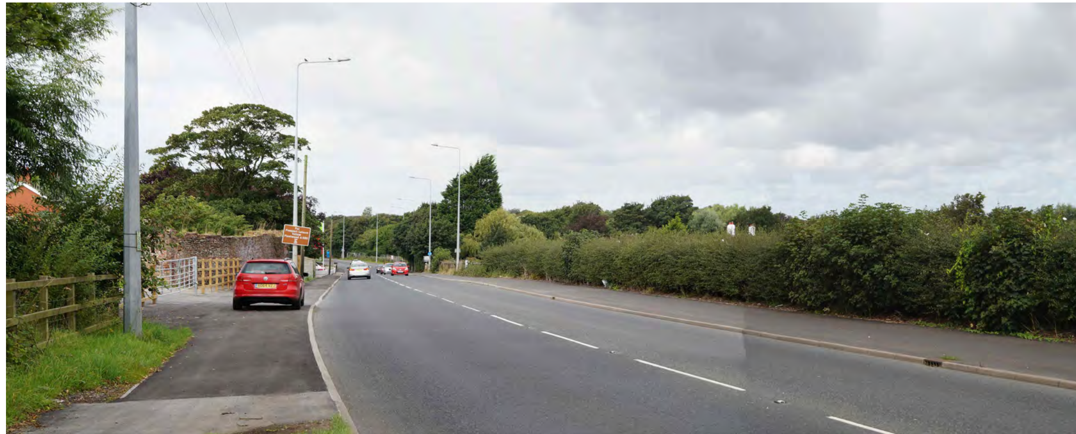
VP6: A585 MAINS LANE LOOKING WEST AND NORTH TOWARDS SKIPPOOL BRIDGE
